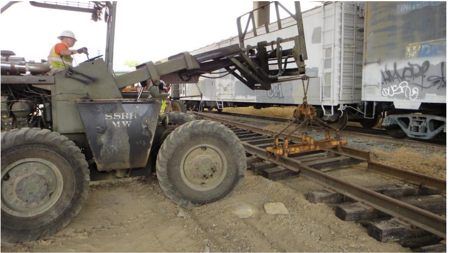
Perfect! Mike T. lining two panels of track together
