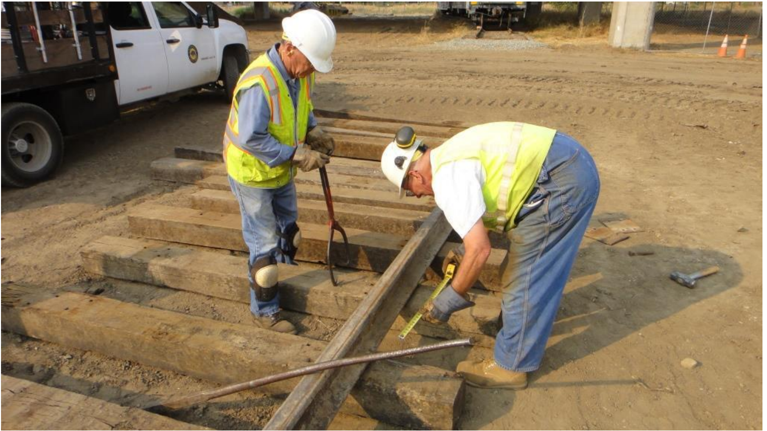
Clem measures the distance between ties as Mike T. lines them the proscribed 24 inches apart
