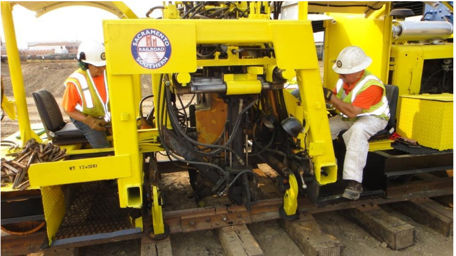
Pam loads spikes into the chute for Mike T. to drive into the ties
