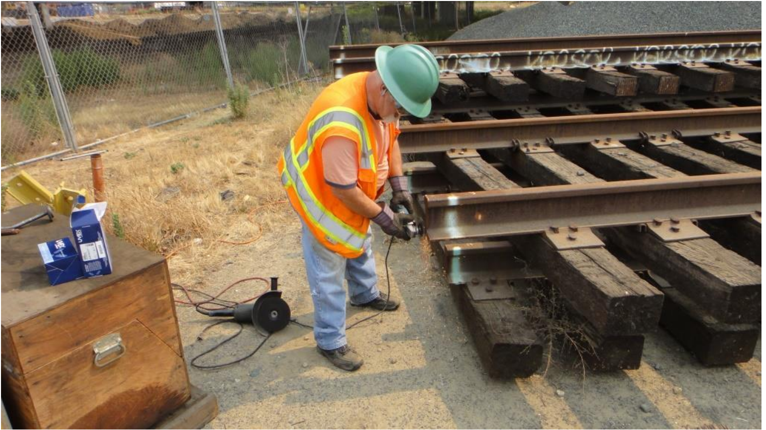
Al grinding the nubs off of the rail-ends
