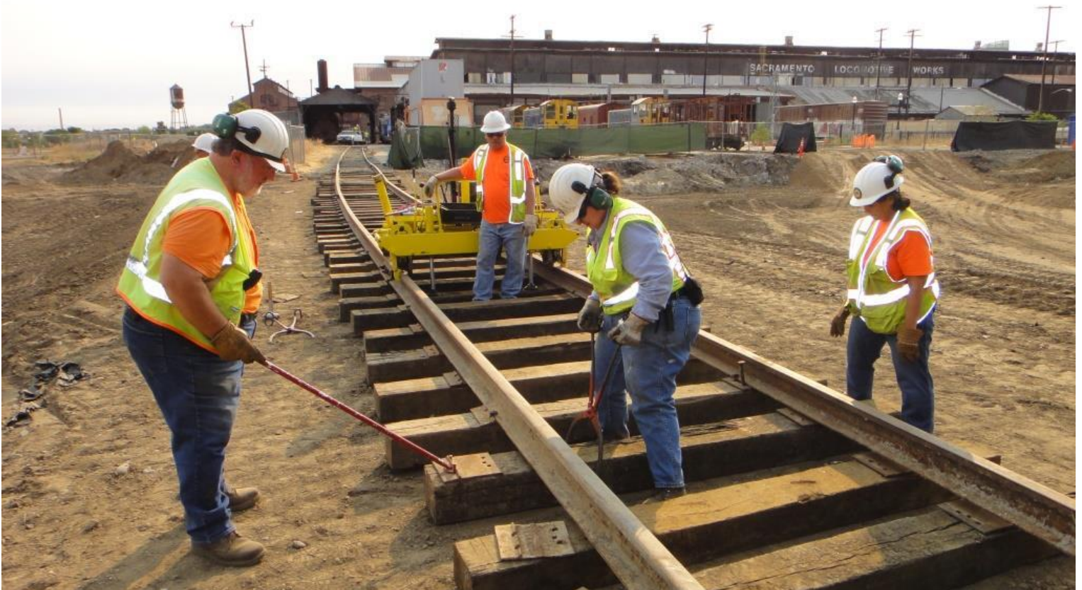
Frank gets ready to insert a tie-plate as Heather and Pam square-up the tie
