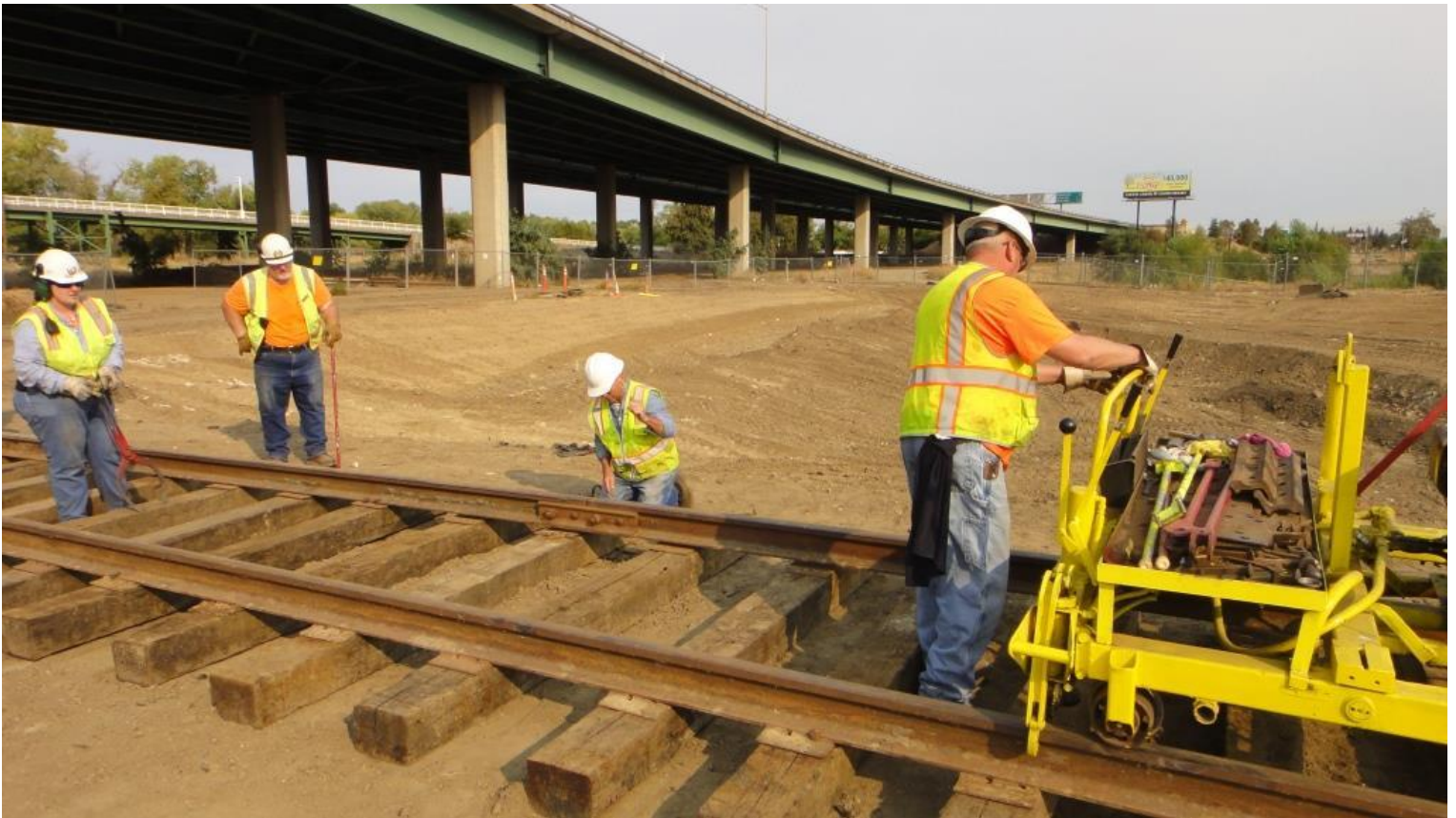
Scott lifts the north rail as Mike T. inserts a joint-plate under the joint
