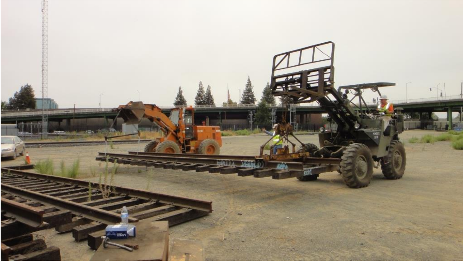
Al in the loader and Mike H. on Big Green lift the panel of track for its move
