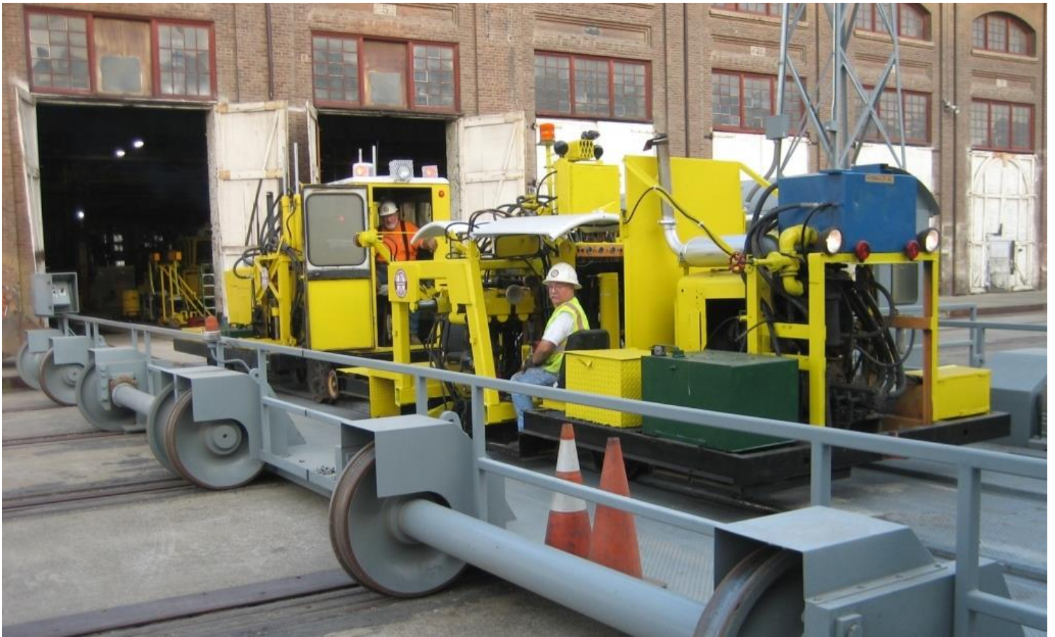
Rearranging the equipment for quick deployment: Frank in the tie-shear and Mike H. in the Super "B" spiker
