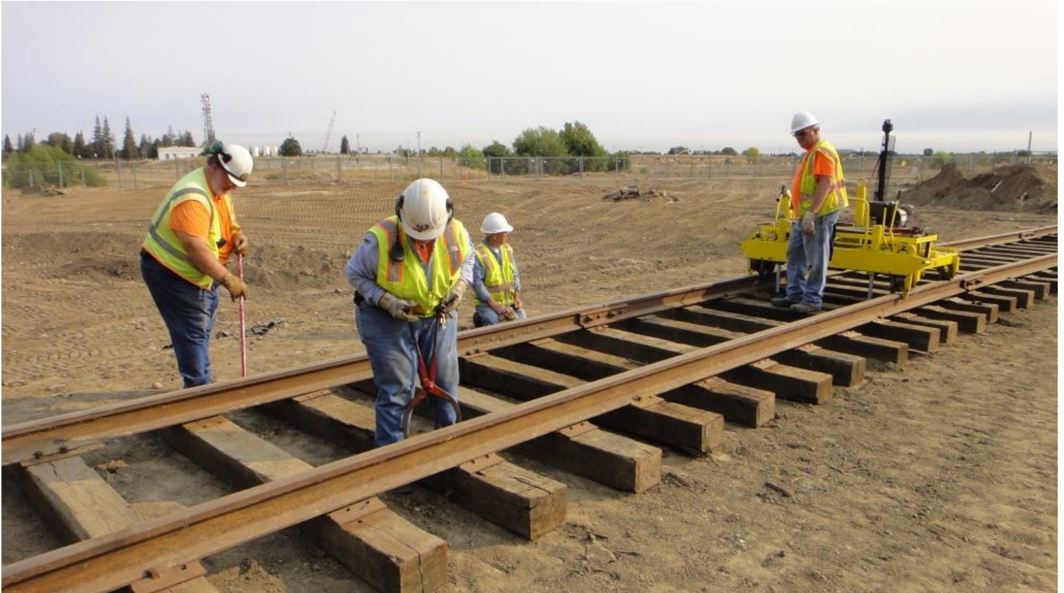
Scott operates the rail-lifter as Frank, Heather, and Mike T. align the ties and insert plates
